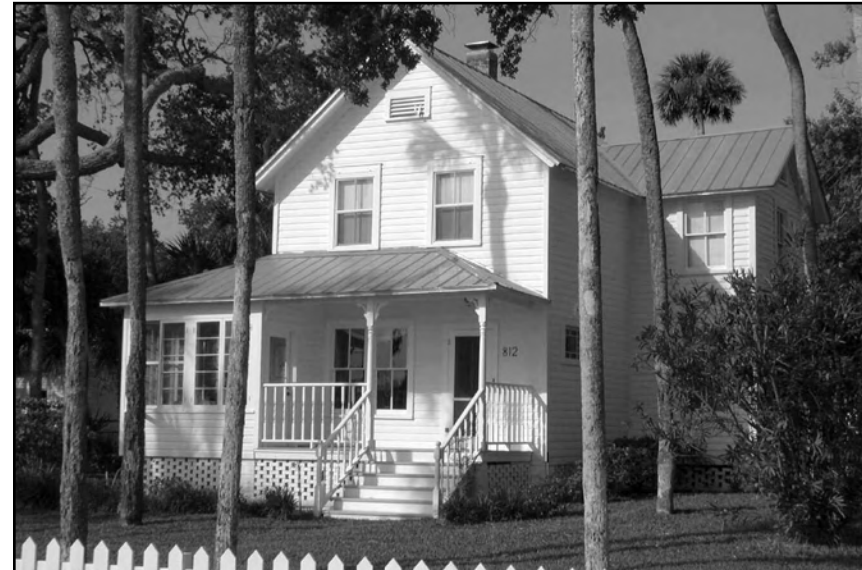
Southern National House with Folk Victorian Railings and Columns
