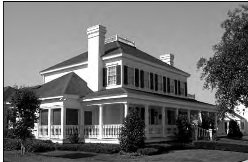
Hipped main body roof
