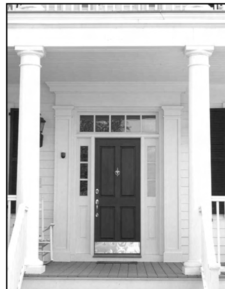
Typical entry condition within a covered porch.
