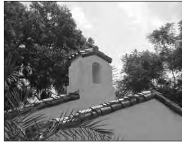
Acceptable alternative chimney detail.
