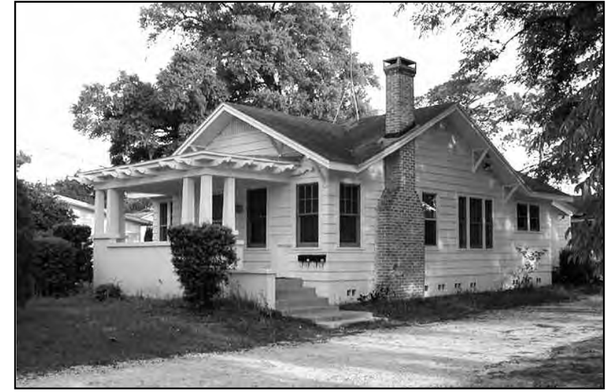
Cross gable with flat add-on porch - Note the triple corner columns and decorative rafter tails.
