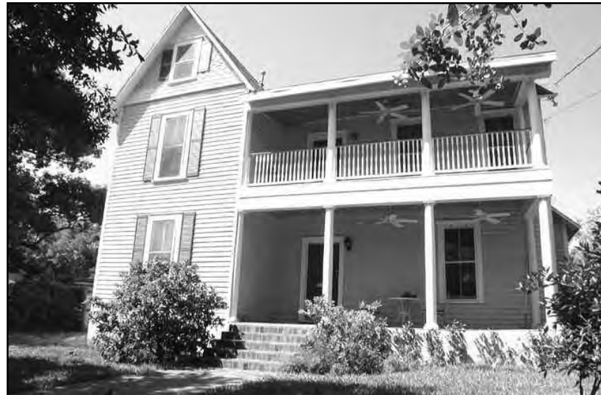
Five bay arrangement with two story porch.
