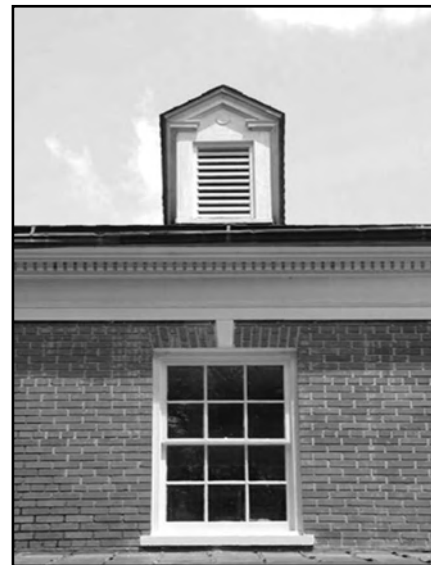
An appropriately sized dormer for ventilation located on a side wing.
