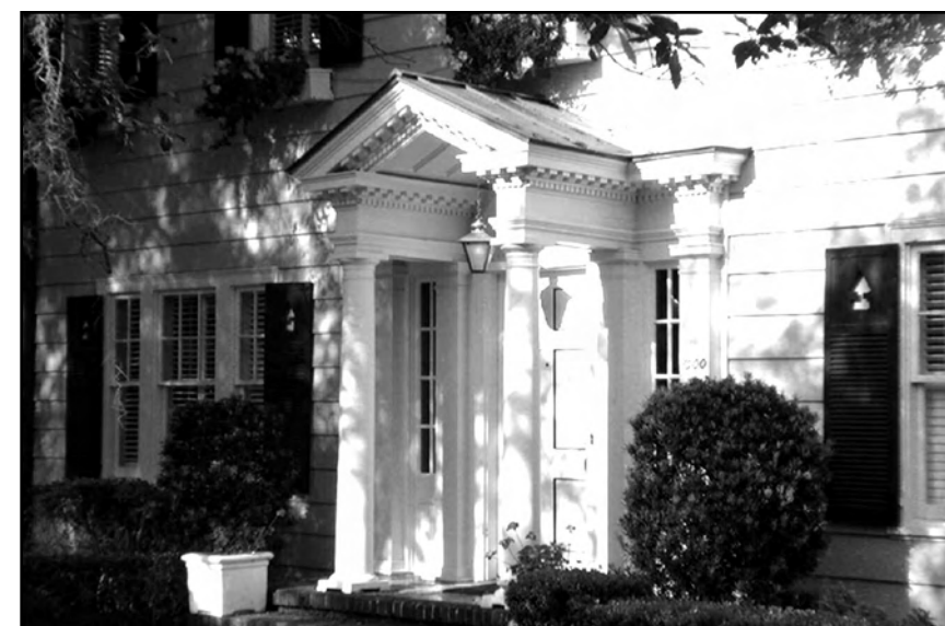
The pediment over the entry is extended out creating a portico for protection from the elements, which is preferable in Orlando.
