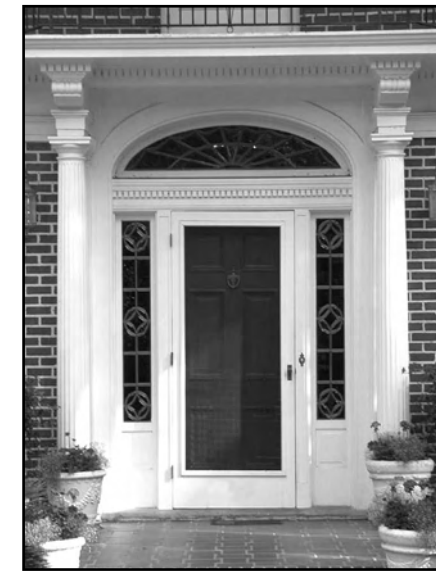
Entry incorporates elliptical fan light and balcony above.
