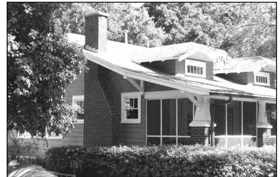
Note hip at end of gable
