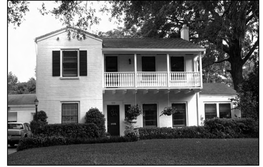
Typical Monterey style. Many homes of this type were constructed of 4" block coursing on both stories, then painted
