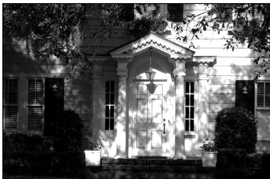
Portico covers entry door only with sidelights encased with pilasters.
