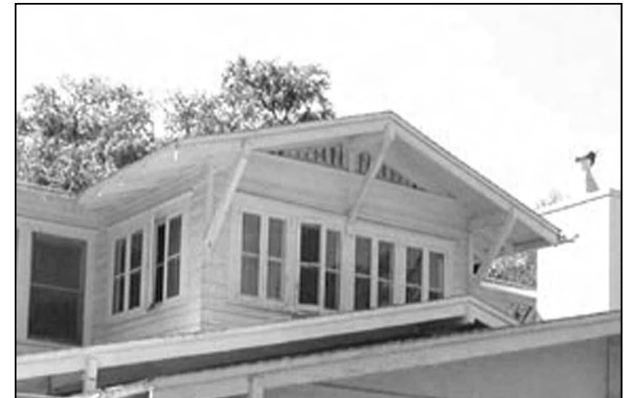
Note the wide decorative gable end vent.
