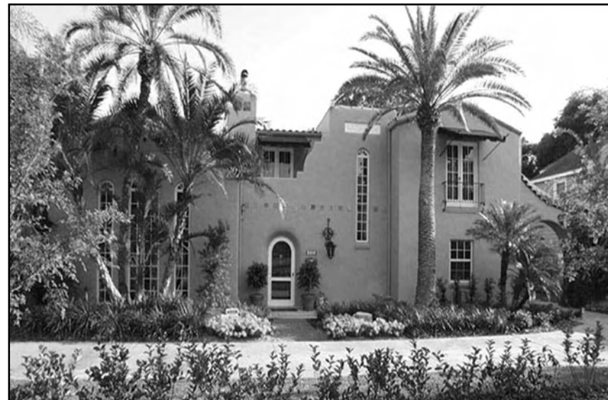
Three distinct bays, the two outside bays have symmetrical window arrangements, the center bay has an asymmetrical arrangement creating points of interest for entry and stair well.
