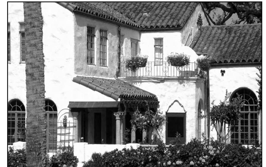
Multiple roof forms, a second story balcony and a loggia provide appropriate massing elements for the Mediterranean style and create a lively street presence.
