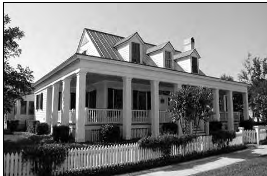
Porch is set behind columns which extend to the ground.
