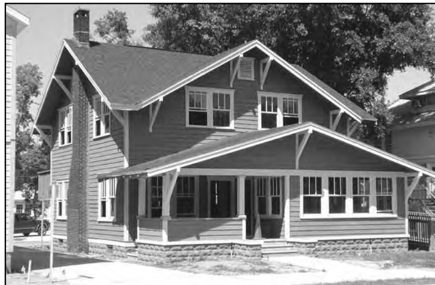
Cross gable 1½ story house. Note the rafter brackets typical of this style.
