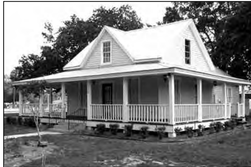
Cross gable roof with full wrapping porch
